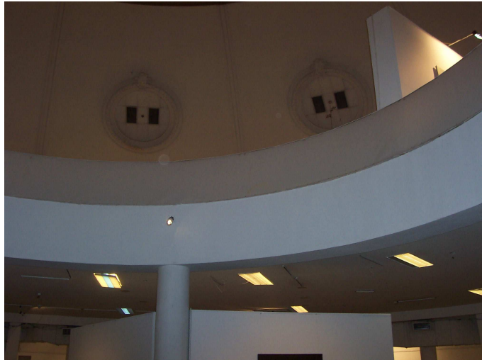
Fig. 8 – Viga circular central s/ P. B
